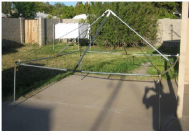
leg with a corner of the pyramid. I used a tee joint in the middle of each wall to attach a sloping roof support, which runs up the middle of each face of the pyramid. This arrangement would make the corners droop, so I added support ropes which run from the peak of the pyramid to its corners. I used bungee cord for these support ropes, but plain rope with a sliding tension-adjustment would work fine too.
